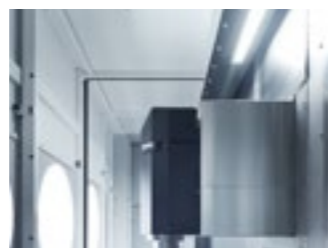
LED lighting in the working area.
